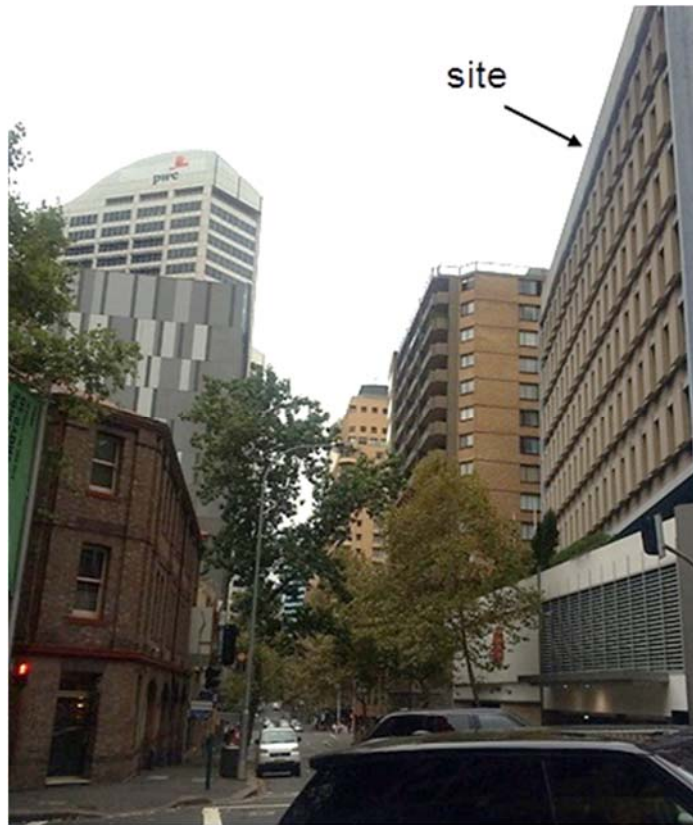
Figure 4: The site as viewed from the intersection of Bathurst and Sussex Streets looking north.
